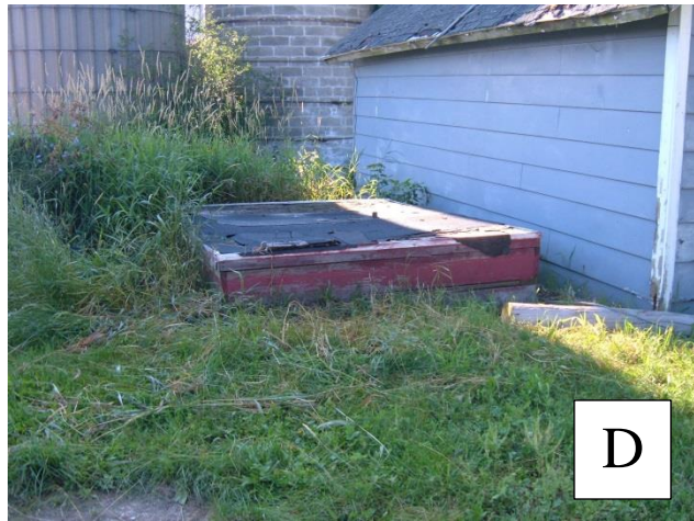
This well pit cover is not structurally sound or watertight.
