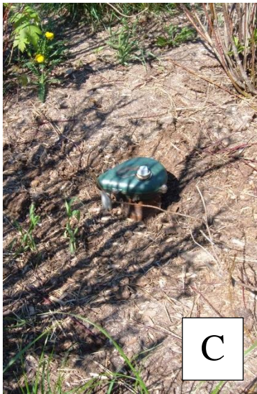
This well cap has been compromised and the well height is less than 8”.
