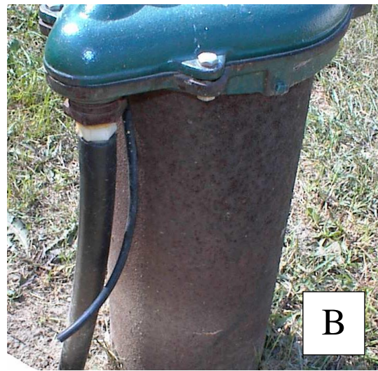
This well cap has a broken o-ring and may have a compromised seal.
